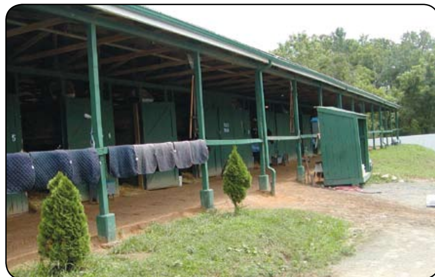
The above horse stable is designed to redirect all roof runoff; a common way to protect clean water from contacting areas that may cause sediment or nutrient runoff.
